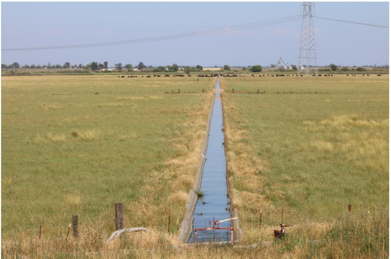
CONCRETE IRRIGATION BITCHES
