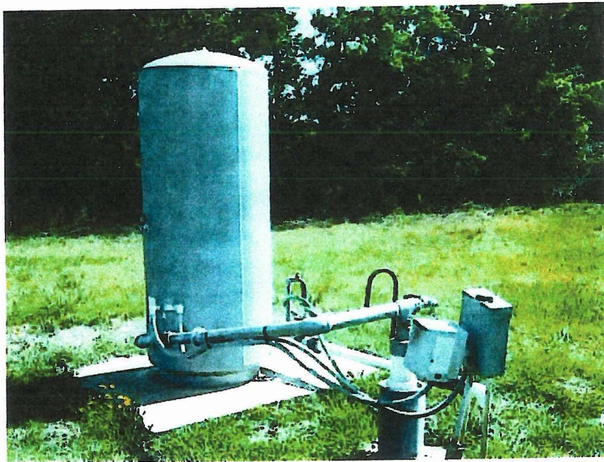
View of 4-inch well
