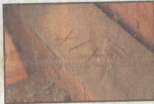
Exposed beams in the loft show Roman numeral markings made when the home was built, which helped the builders construct the home.
