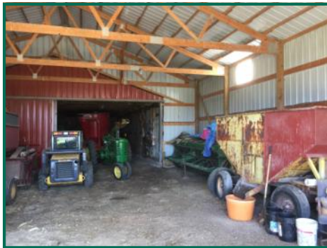
Steel Utility Building 32' x 40' built in 1978.
