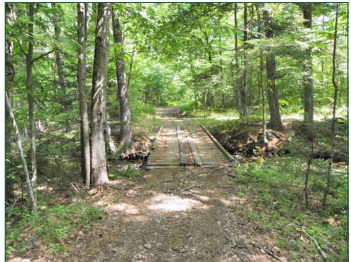
The Pease Brook bridge can support vehicular traffic but the decking will need repair soon.
