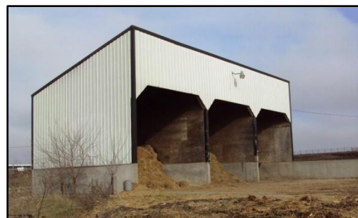
Commodity Shed on Tract # 1 at Feed lot Concrete bays & Apron
