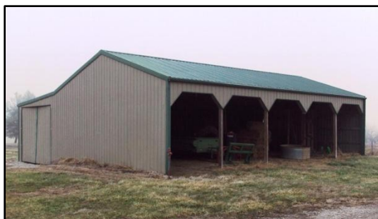
Machinery Shed on Tract # 1 Metal with wood frame
