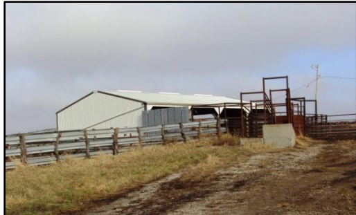
Working Barn, Corrals & Load Out at Feedlot Guard Rail & Steel Corrals, Working area w/chute
