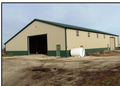
7,000 sq ft Barn on Tract # 1 2 – 14 x 20 ft Overhead doors & Elec. Lifts, concrete apron,
