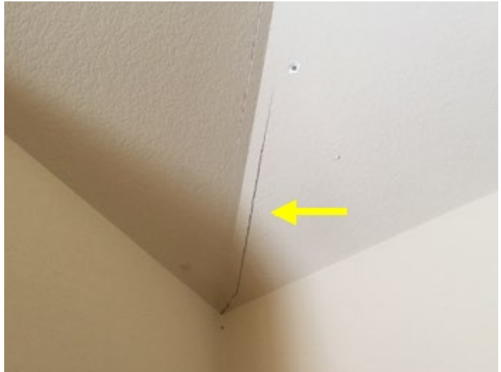
Crack observed to ceiling in master bedroom.
