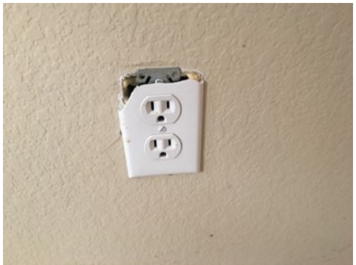
Damaged faceplate present at outlet in breakfast nook.
