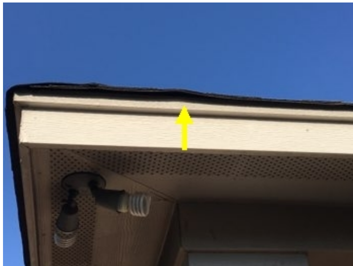
Missing drip edge flashing.
