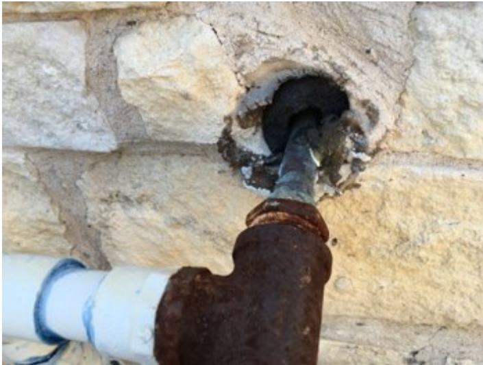
Exterior gas line on the right side of the home is not properly sealed with siding materials.
