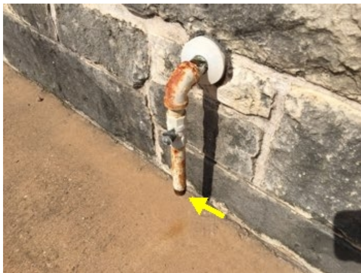
Recommend adding a nipple (cap) to exterior gas line at the back side of the home.
