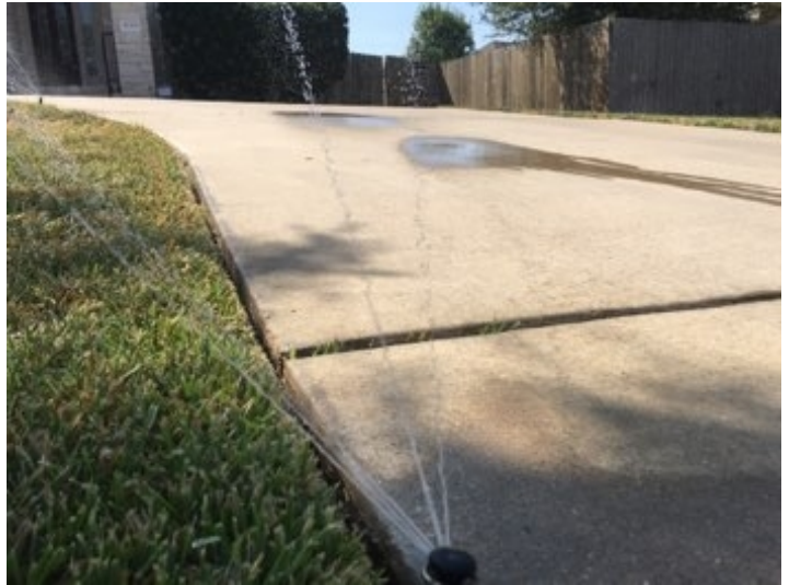
Zone 1 sprinkler head at front corner of yard spraying against driveway. Recommend adjustment
