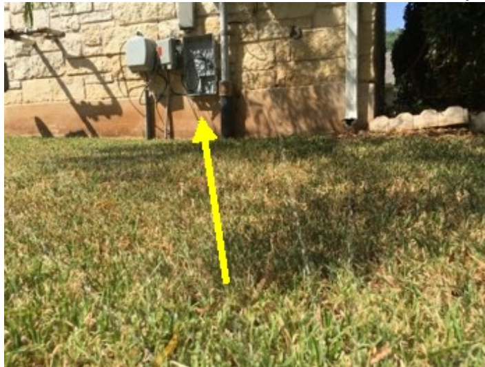
Zone 1 sprinkler head at left side of yard spraying against cable equipment/ electrical panel and home. Recommend adjustment.
