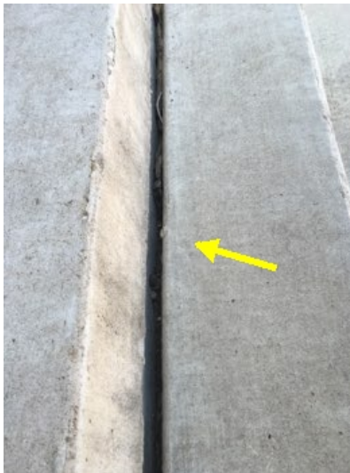
Deterioration observed to wooden joint at front entry stairs. Recommend sealing to prevent water penetration.
