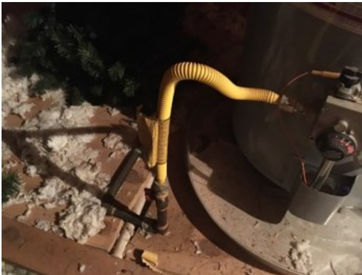
Missing drip leg to gas line.
