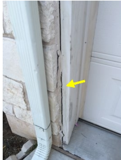
Exterior garage trim is not properly sealed. Recommend sealing to prevent pest and water intrusion.
