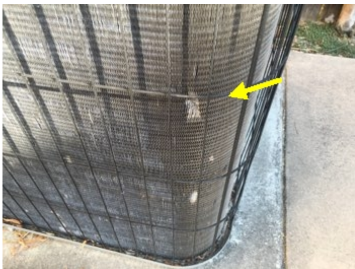
Hail damage present to exterior condensing unit fins.
