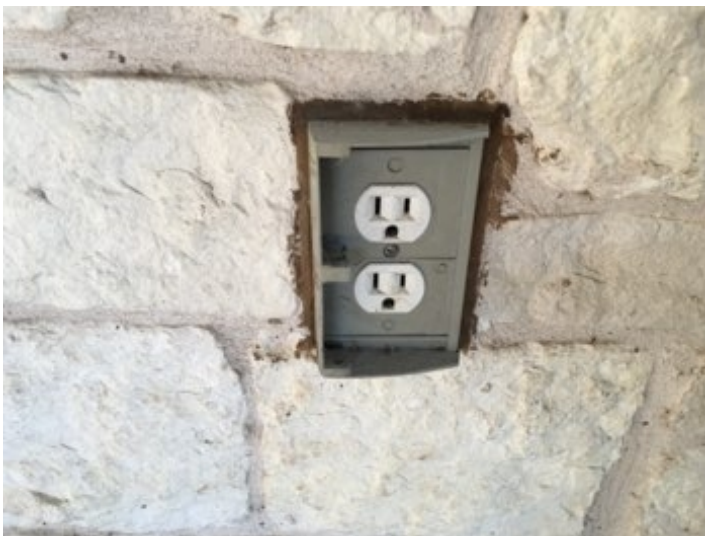
Exterior outlet at back patio missing cover
