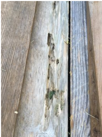
Wood located directly against structure. Evidence of wood destroying insects (Termites) present in wood.
