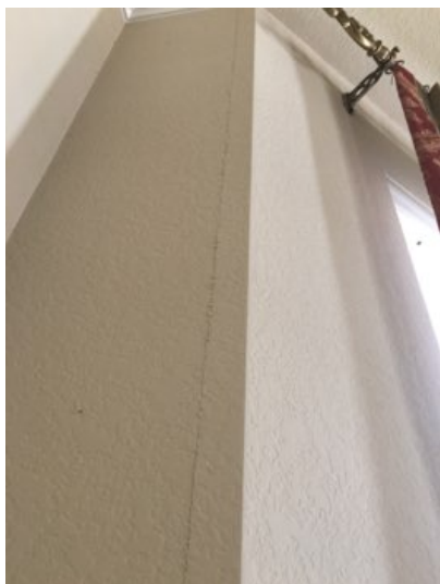
Crack observed to interior wall in breakfast nook.
