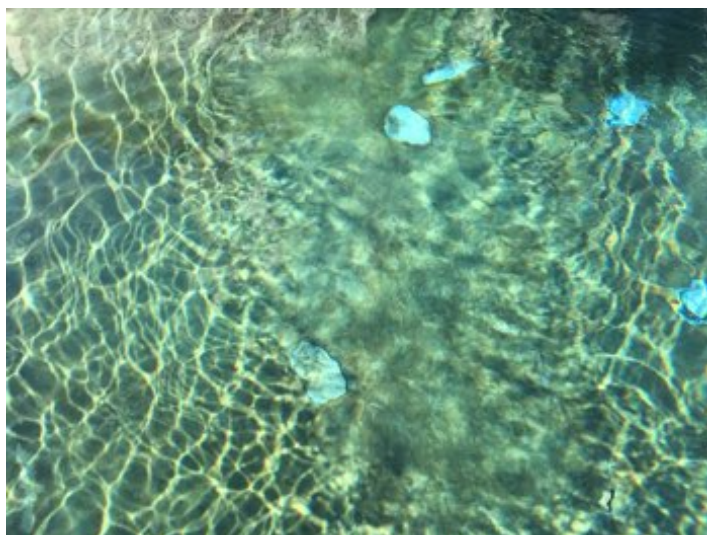
Deterioration observed to topcoat at base of pool and spa. Recommend evaluation from a licensed pool specialist.
