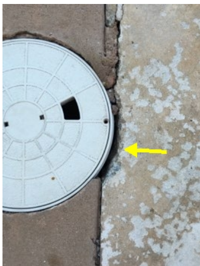
Gap observed to sealant around drain. Recommend sealing all gaps in pool decking to prevent water intrusion.
