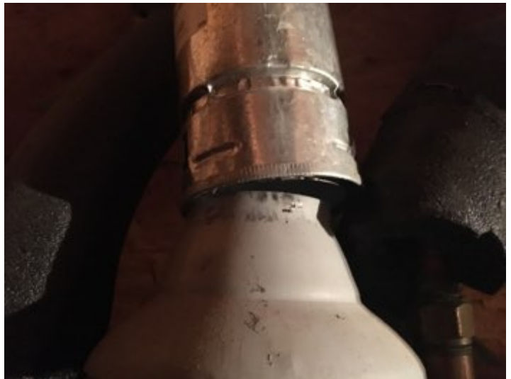
Water heater vent not properly attached. Vent is melting insulation located too close to termination point.
