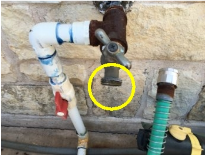
Missing backflow preventer on exterior water spigot at he back right side of the home.
