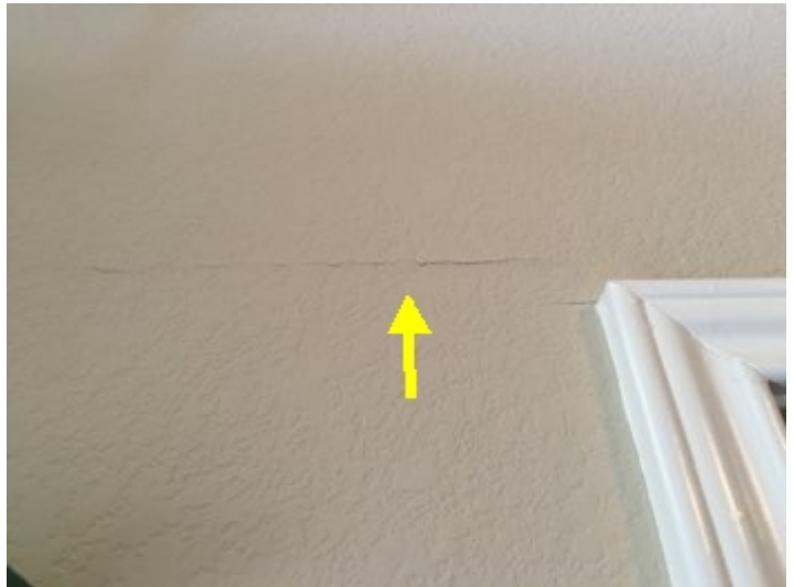
Crack observed to interior wall above french doors leading to front living area.
