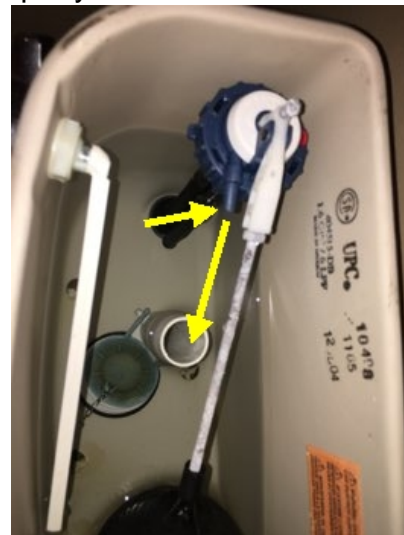
Toilet assembly in hallway full bathroom is missing its fill tube.
