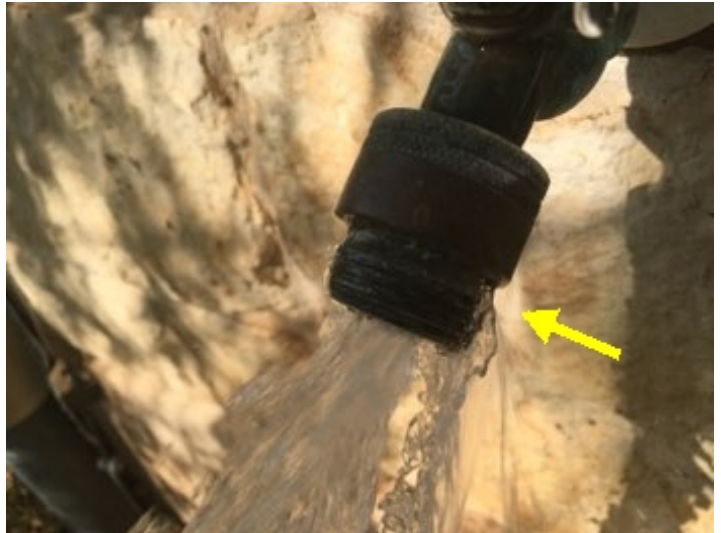
Hose bib at front left side of the home leaking around the back flow prevention. Hose bib is not properly sealed with exterior wall.
