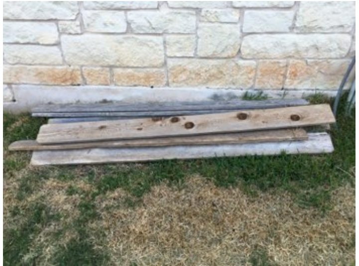
Wood located directly against structure. Recommend storing unused wood away from the home. Evidence of wood destroying insects present in wood.
