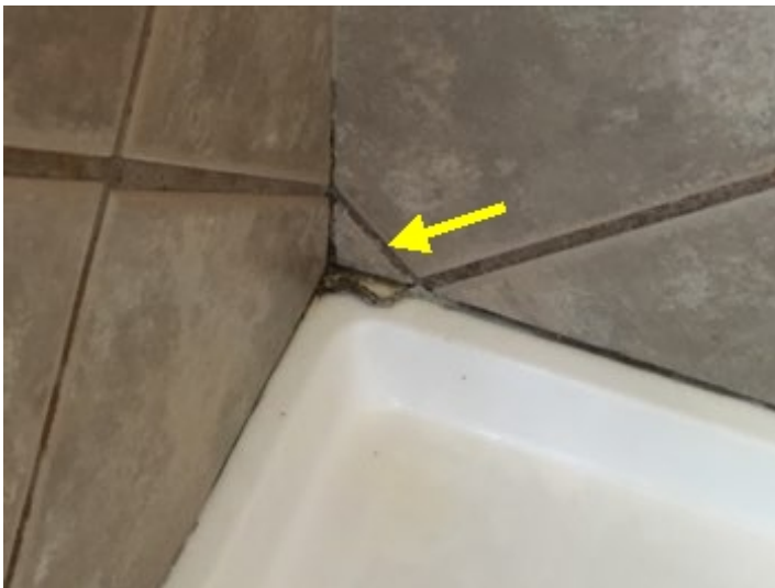
Deteriorated sealant present at master bathroom shower enclosure.
