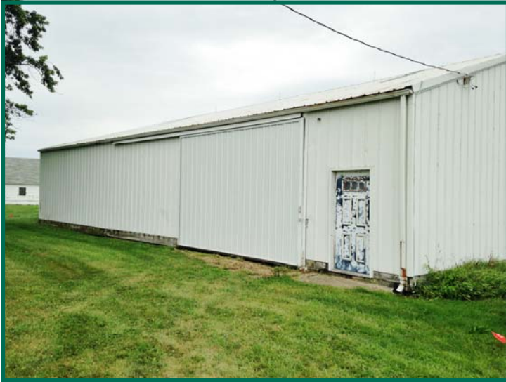
64' x 42' post frame shed
