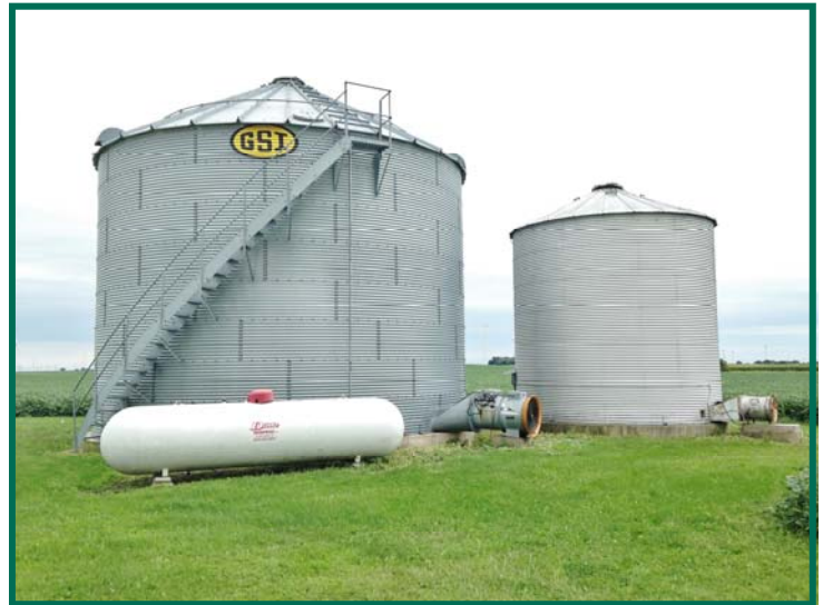
30' x 8 ring bin with drying equip. (left) & 18' x 6 ring bin (right)
