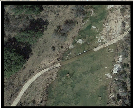
Concrete River Xing
