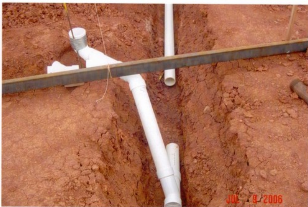
plumbing before concrete
