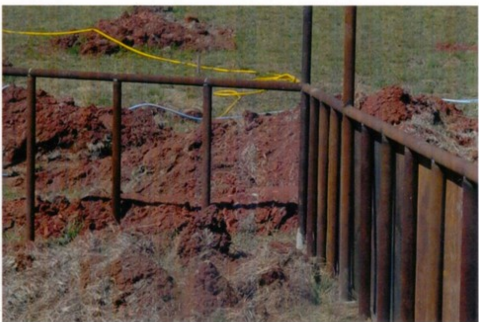
building a retaining wall
