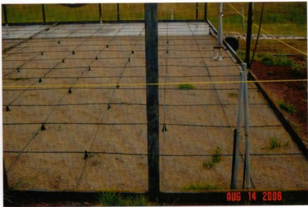
lots of rebar
