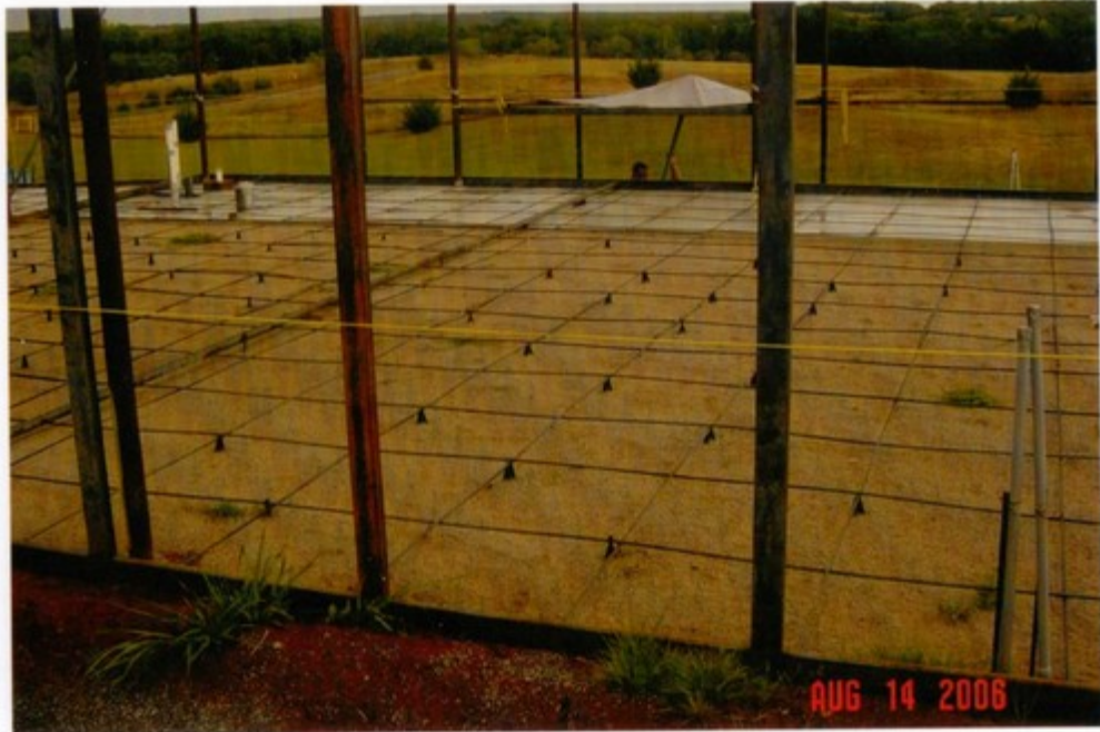
lots of rebar
