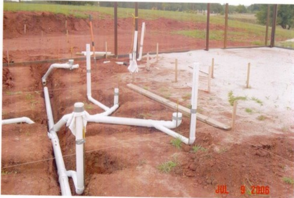
plumbing before concrete
