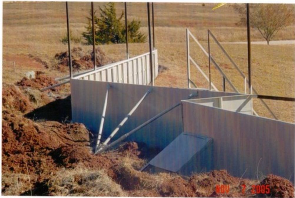
more retaining walls
