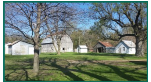
All of outbuildings located behind dwelling.
