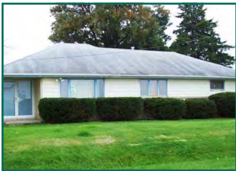
2nd View of 13741 N 71st Ave W
