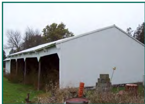
Open Front Shed
