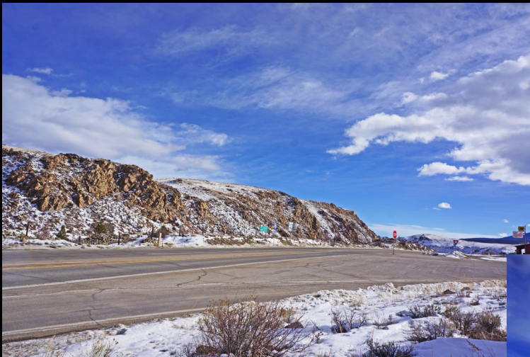
Highway View South
