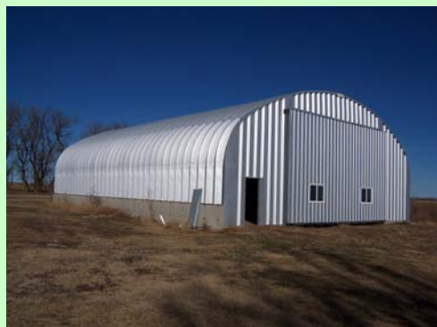
Tract 3 Quonset Building
