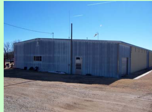
Tract 4 Shop Building
