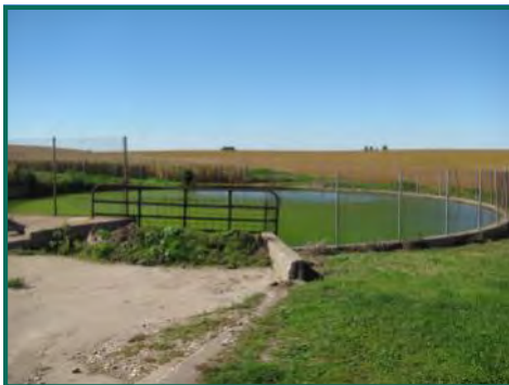
Concrete Manure Pit
