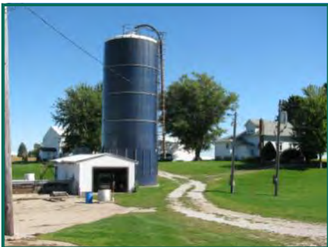
Silo and Machine Shed
