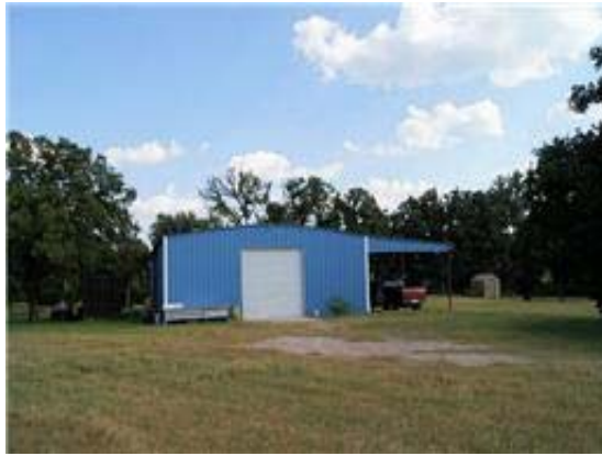
2400 SF Metal building w / 20' Shed attached on west side of building
