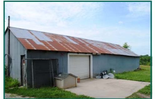
Parcel 2 - Machine Shed (Overhead Door)
