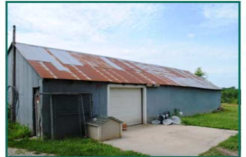
Parcel 2 - Machine Shed (Overhead Door)
