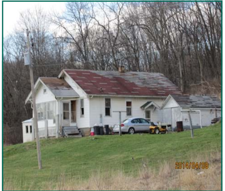
View of house looking south-west.
