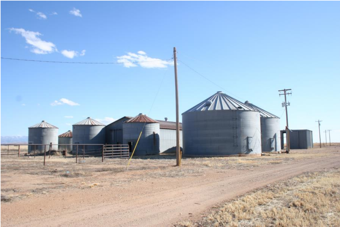
Grain Storage bins approximately 40,000 bu. capacity
