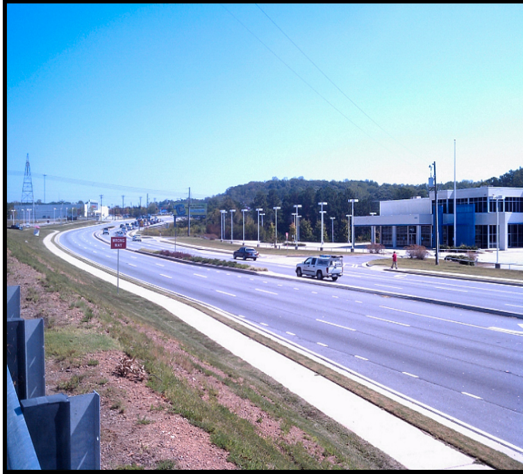
HIGHWAY 78 FACING EAST
