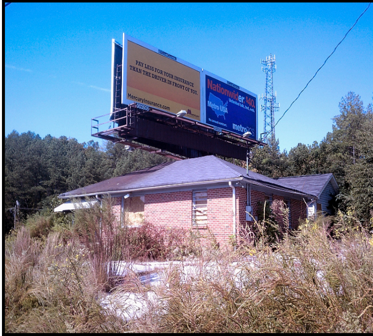
HOUSE, BILLBOARD AND CELL TOWER ON SITE
