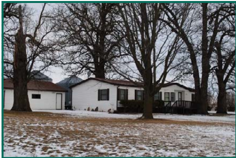
House - Built 1987, Garage - Built 1996
