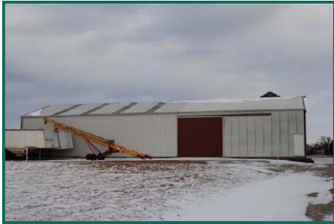
4,000 SF Machine Shed - Parcel 1
