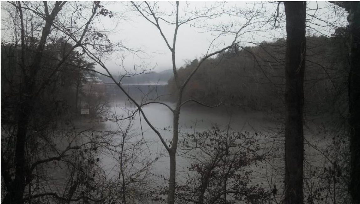
View of Lake Yonah Dam
