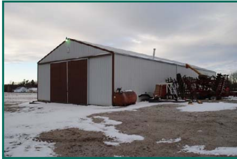
Machine Shed - Parcel 1
