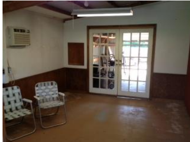
Office with Air Conditioning
