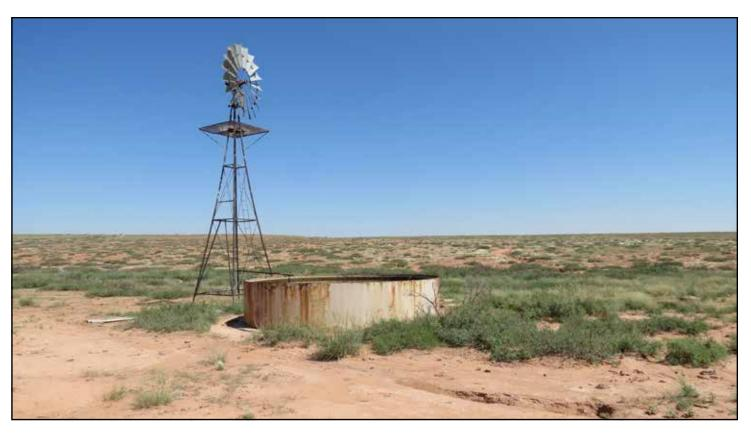
The operating windmill is located on the east side of the ranch. This well is located along Wylie Draw. It is equipped with an electric submersible pump, and a portable generator is used to pump this well when the wind is not blowing. This portable generator will stay with the property.
