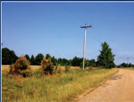
County Road #108 Frontage
