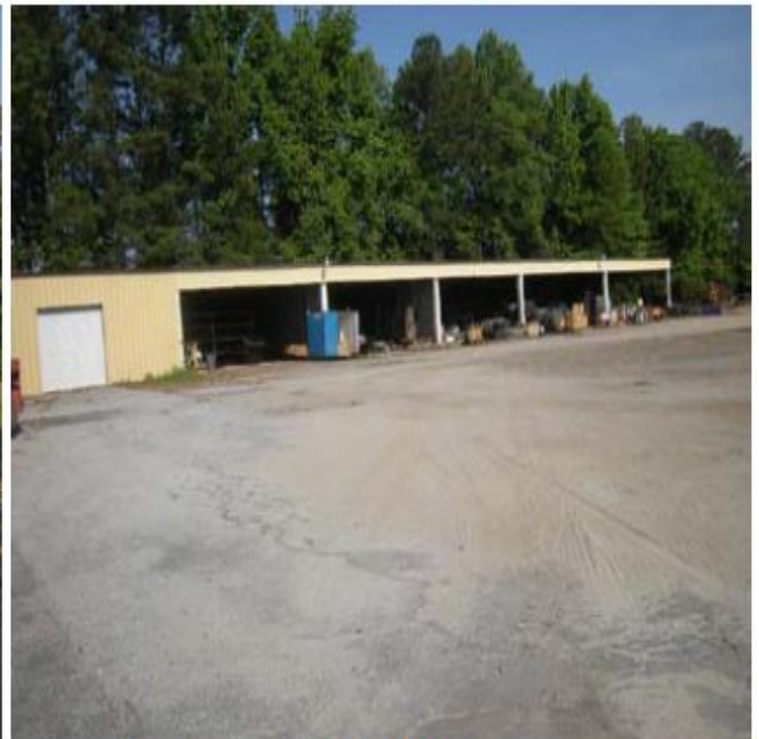
View of Shed Building
