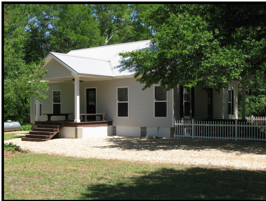
Side View of Home and Yard
