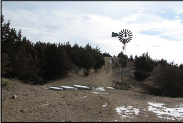
South water site with windmill, three tanks & submersible well
