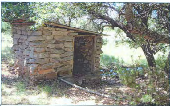
Old Structure Built over Spring
