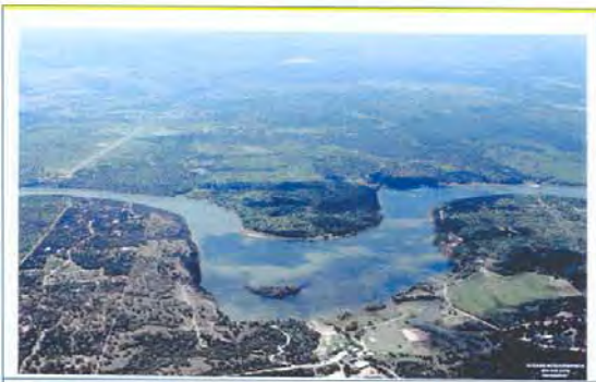
Arial View to the South
