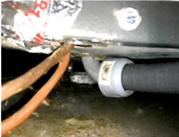
replaced uninsulated wires to AC / heat pan with new, insulated wiring
