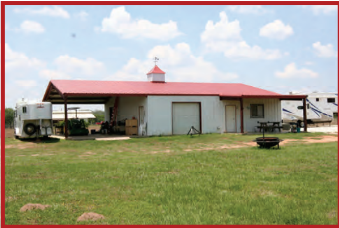
Multi Use Building
