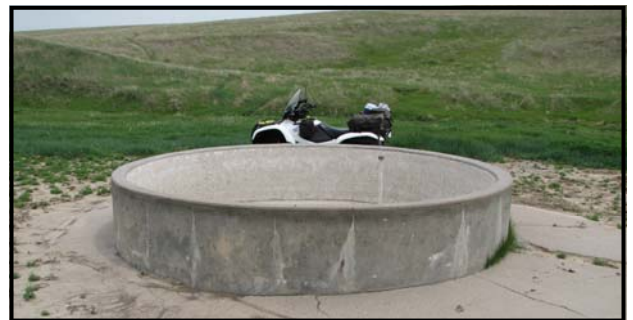
Concrete tank with pad on pipeline
