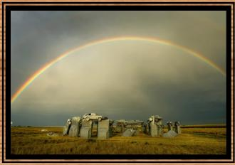
sume the same proportions as Stonehenge with the circle measuring approximately 96 feet in diameter. Some autos are held upright in pits five feet deep, trunk end down, while those cars which are placed to form the arches have been welded in place. All are covered with gray spray paint. The honor of depicting the heel stone goes to a 1962 Caddy.
