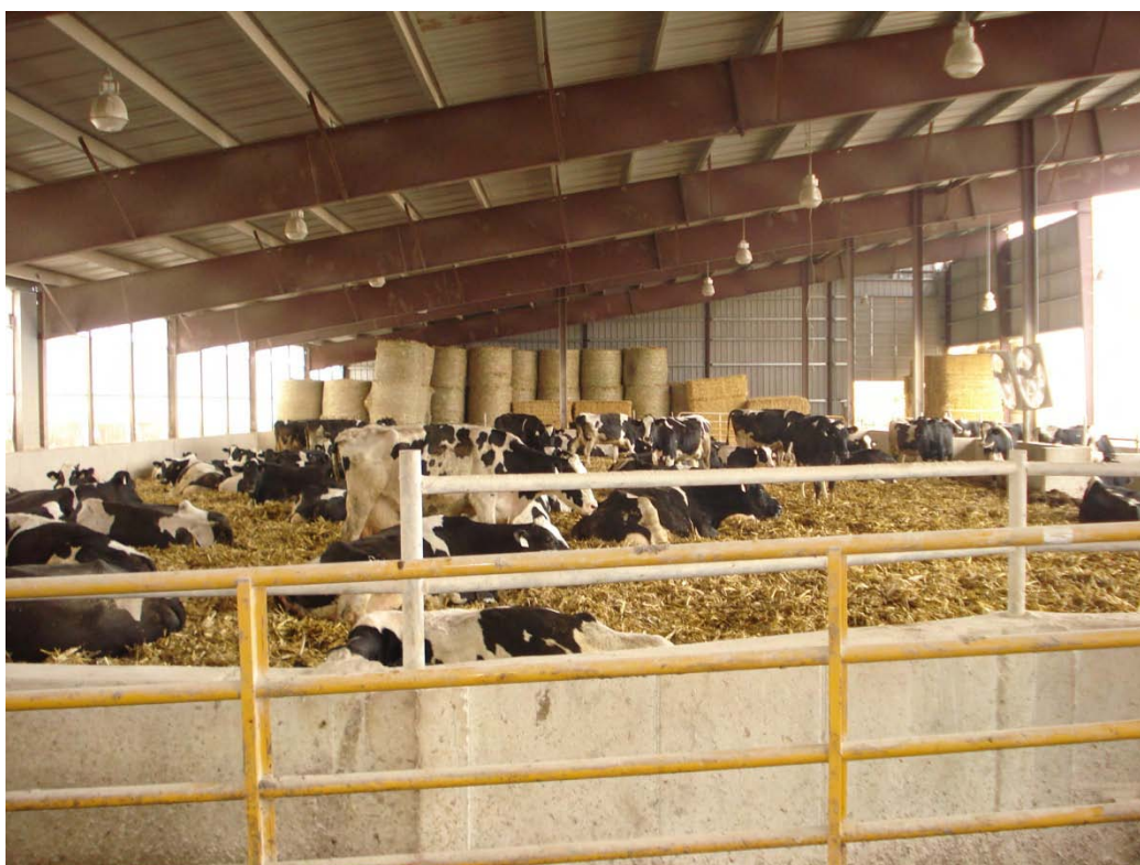
Bed Pack System with cement manure storage
