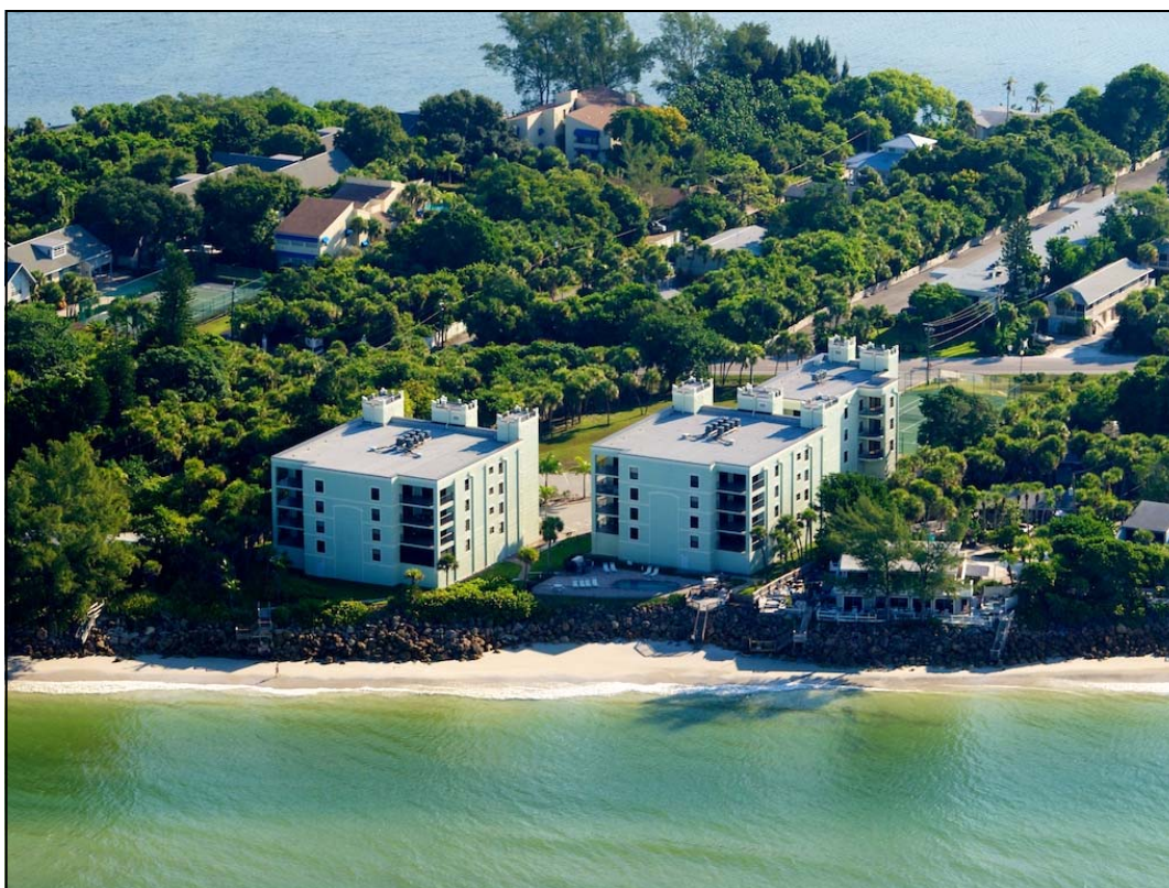
Boulder Point Condominiums, North Beach Road, Manasota Key, Englewood, Florida
