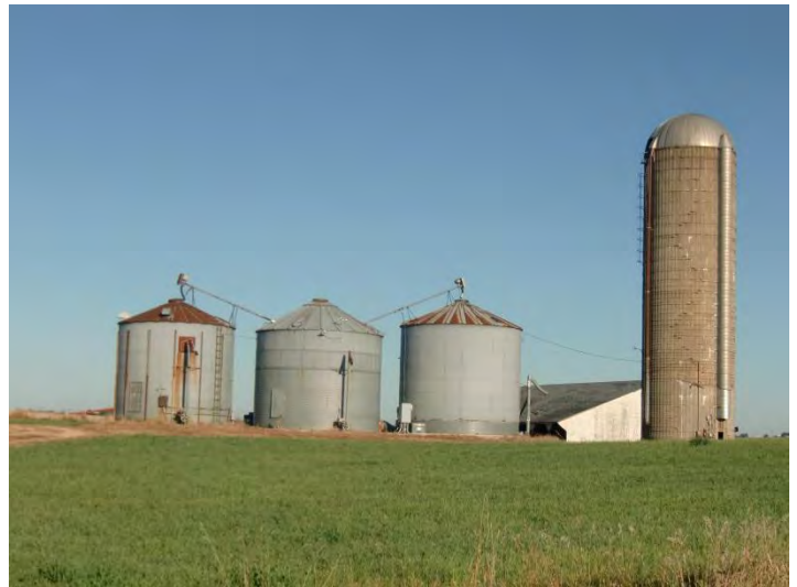
Parcel #2 – Grain Bins & Silo
