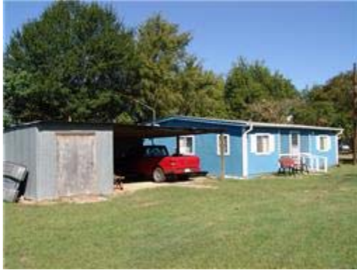
Frame home & carport
