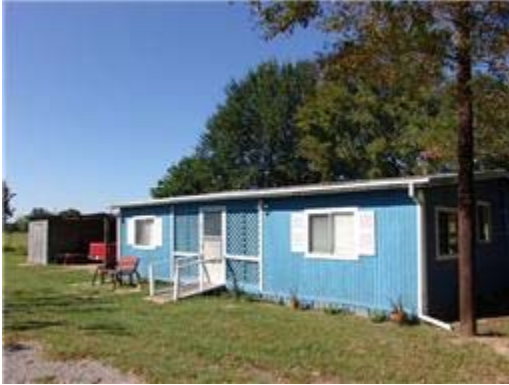
Front view of frame home
