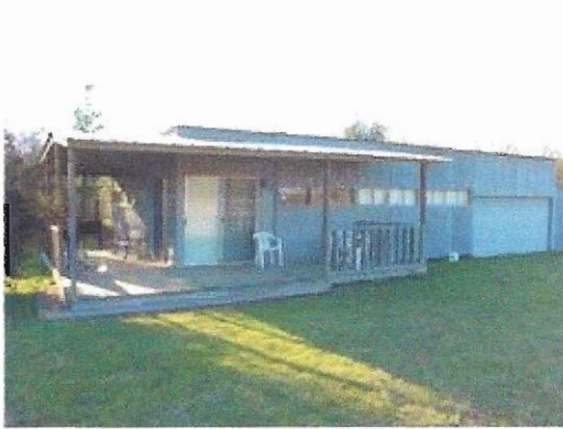
Front view of cabin
