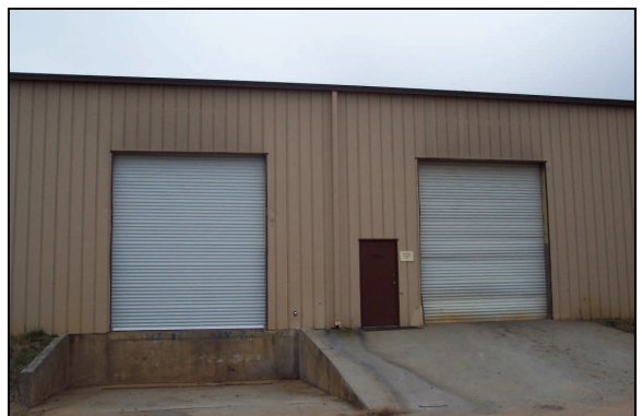
Dock High and Drive In Doors
