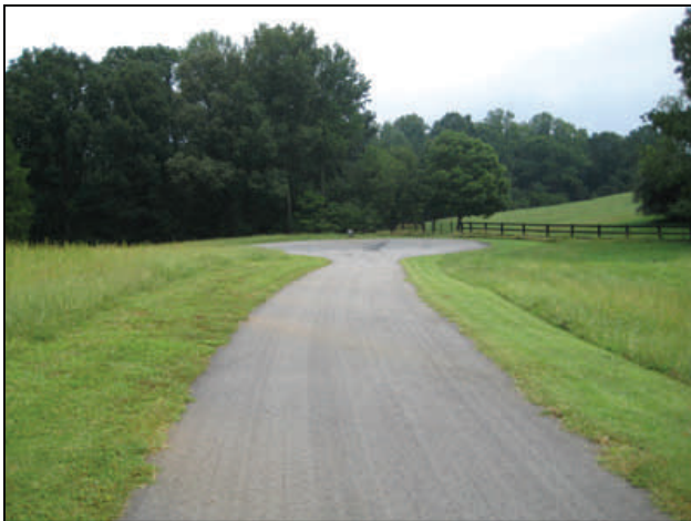
Paved interior road system
