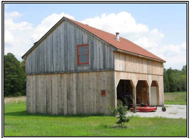
VIEW OF BARN FROM THE NORTH
