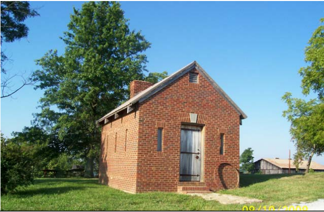
ABOVE: The Brick Storage Building. It far exceeds that of a typical storage building, and is more like a small (12' x 16') shop. It is of solid brick construction, with concrete floor, with fireplace, and "gun-port" style windows, and insulated wood door with blacksmith ironwork!
