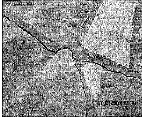
Mortar crack in stone on right side of entry.
