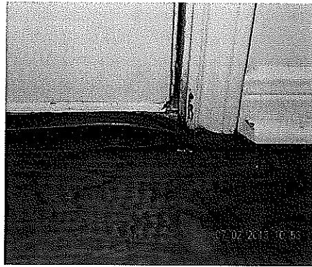
Evidence of water penetration on the floor at the back door in master suite.
