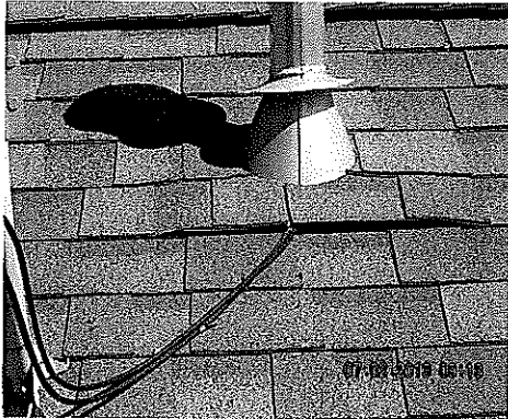
Satellite dish cable has roof jack kicked up at water heater vent pipe.
