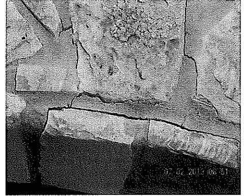
Mortar crack in stone on front of entry.
