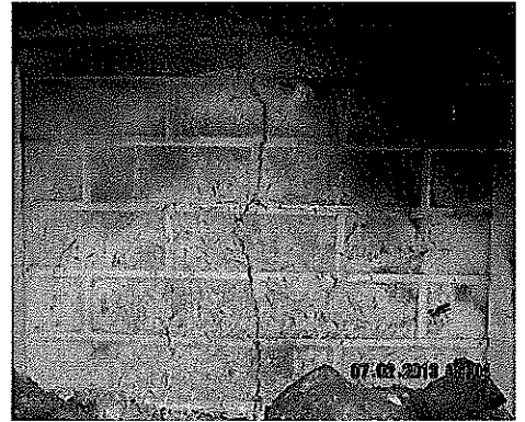
Crack in back of both fireplace fireboxes.
