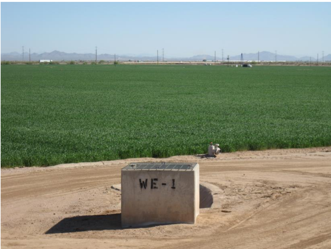
MSIDD irrigation water turn-out
