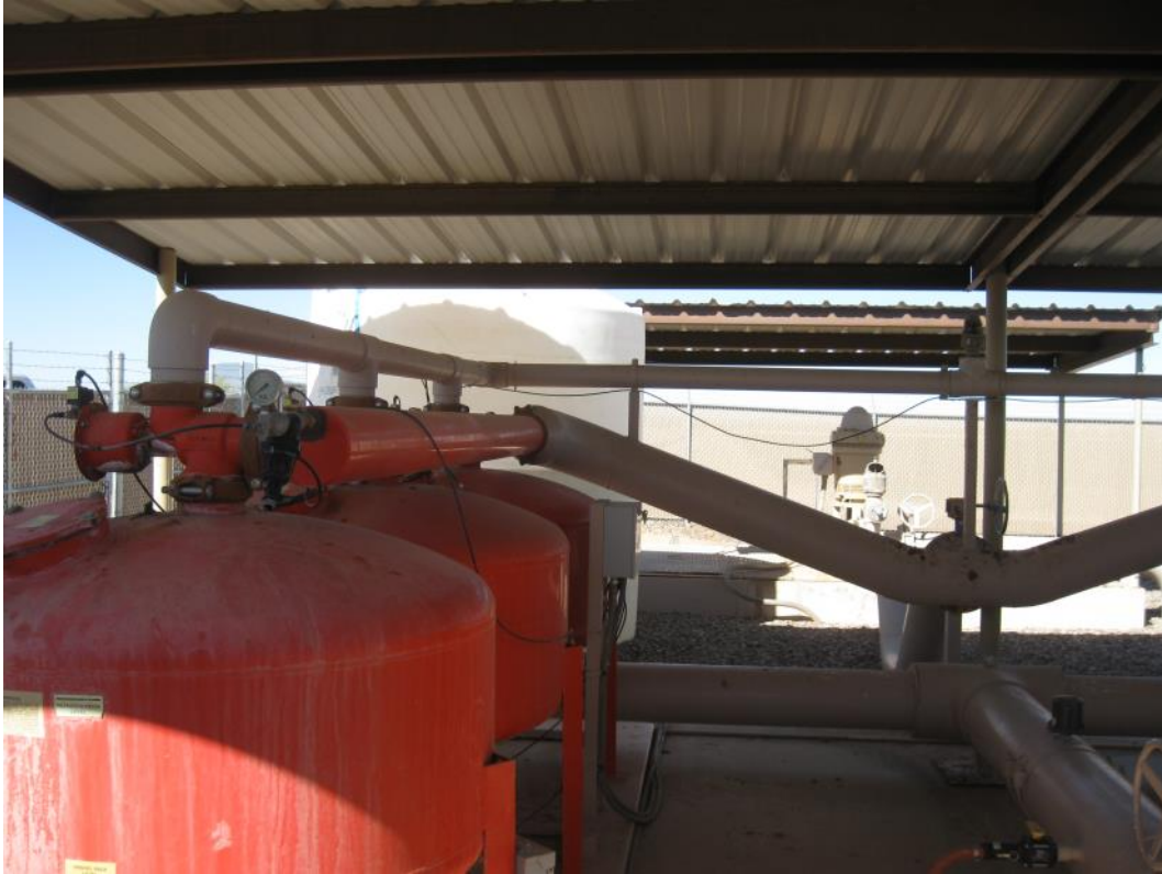
Drip irrigation sand media filters
