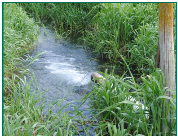
Sump Pump Outlet
