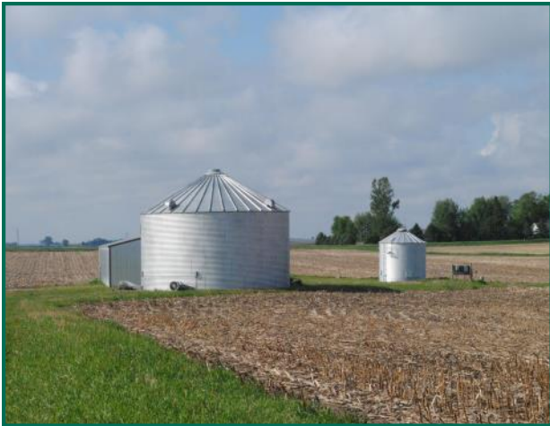
Building Site - Corn and Soybean Storage Bins
