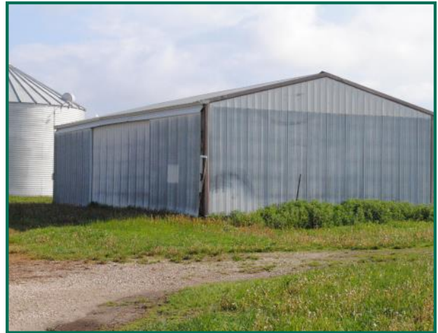
Pole Building - New Roof Spring 2017
