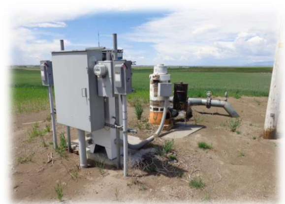
Looking west at the well in the SE, Section 11. 200 hp, GE motor & Layne bowler turnine pump.
