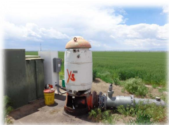
Pump in the NE of Section 02. 150 hp, Worthington ump, US motor.
